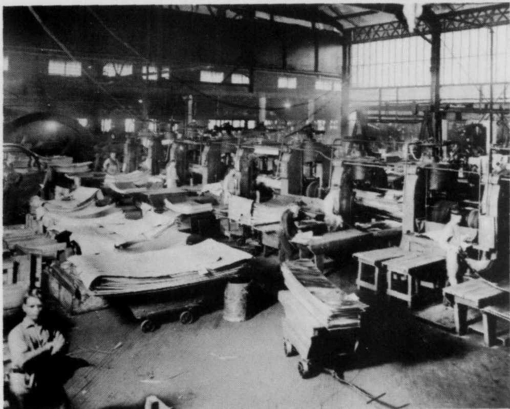
In 1912, Alcoa's New Kensington Works boasted the latest technology in flat sheet rolling mills. Two men worked at each station "man-handling" the sheet back and forth through the rollers.
