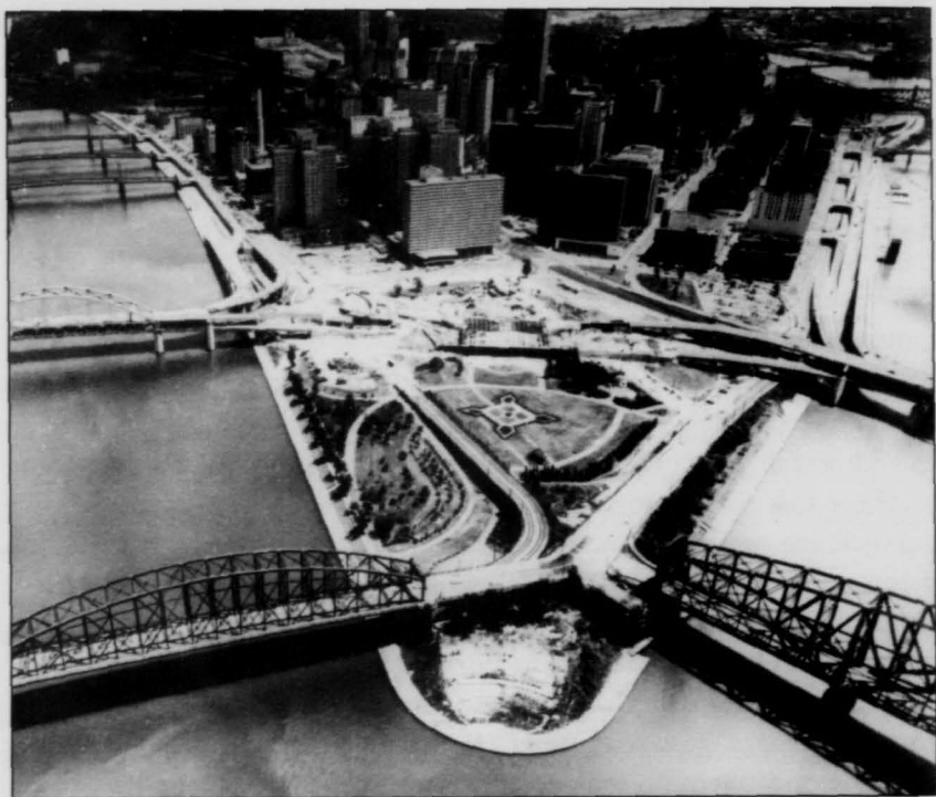
This early 1960's view of the construction of Point State Park shows both the old point bridges and the new ones still under construction. The old bridges had to be replaced with new ones farther from the point for the park's design to work.
