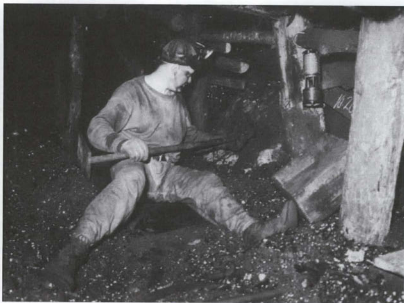
FIGURE 7 Joe Gladski, miner, setting dynamite in tunnel 29 in Maple Hill mine. Seldon Dick 1938
