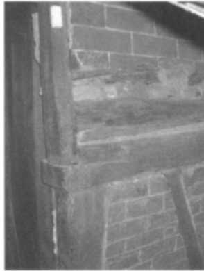
Figure 3: Former exterior wall, Gemberling-Rex House. This wall, now accessible in the uppermost portion of an eighteenth-century addition to the building, shows the early exterior finish of the structure. The timber framing was filled, and the infill was plastered, scored, and painted to resemble brickwork. Photo, Diane Wenger, 2007.
