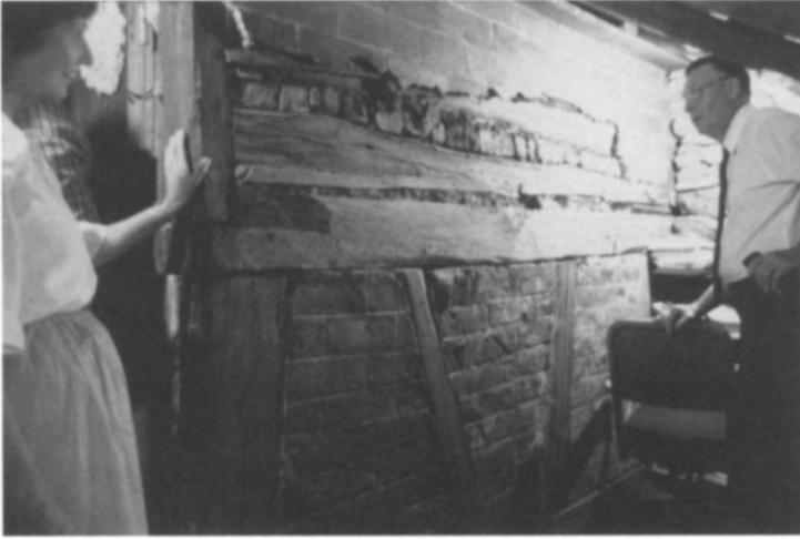
Figure 10: Gemberling-Rex House, lean-to attic, showing the three logs added above the original fachwerk. Photo by the author. At the extreme right is Robert C. Bucher, author of many seminal articles on Pennsylvania German architecture. This article is dedicated to him.
