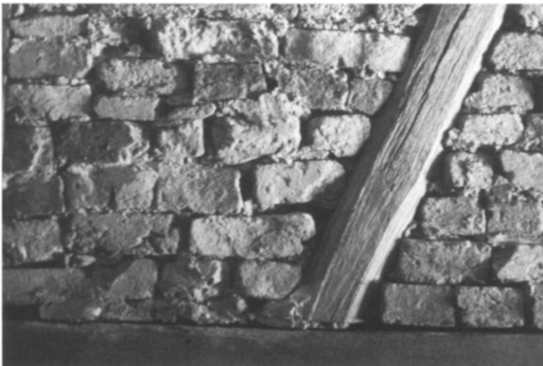
Figure 5: Gemberling-Rex House lean-to attic, showing the original exterior rear wall, with exposed, unfinished nogging, indicating a very early lean-to shed addition. Photo by the author.
