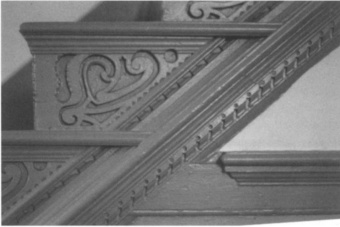
Figure 20: Jig-cut end blocks of the rear-facing durchgangigen stair, a spectacular example of vernacular Rococo. Photo by the author.
