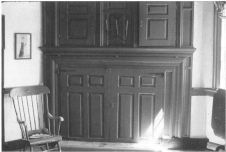
Figure 17: the front parlor, showing the ill-fitting fielded panels. Photo by the author.
