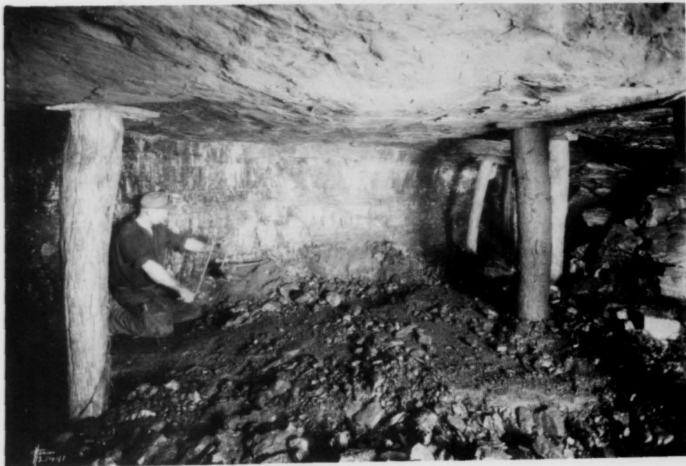
Photo of mine worker drilling at "low coal" (1925).
