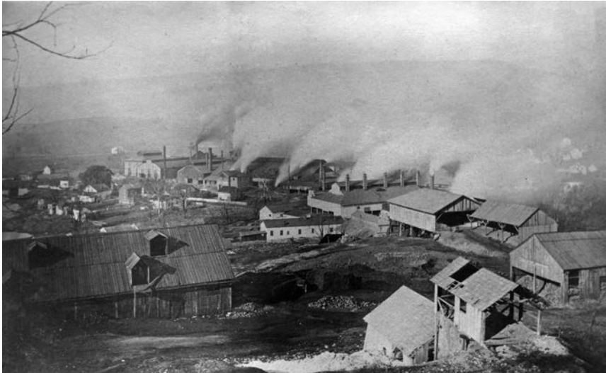
FIGURE 7 Overview image of Standard Steel and Logan Iron and Steel, circa 1880. Standard occupied the two stone buildings to left of center at this time. These were originally built for the Bessemer plant in 1868. Next was the hammer shop, rolling mill, tire mill, and forges (with the five chimneys in a row) of Logan Iron. In the bottom right and foreground are the structures associated with Emma Furnace. Courtesy of the author’s collection.
