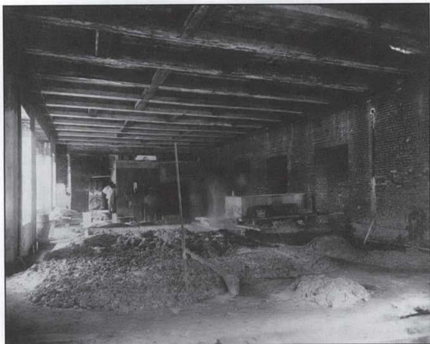
Fig. 12. Mixing and pouring concrete floor at HSP. Photo by C. S. Bradford, September 27, 1906.
