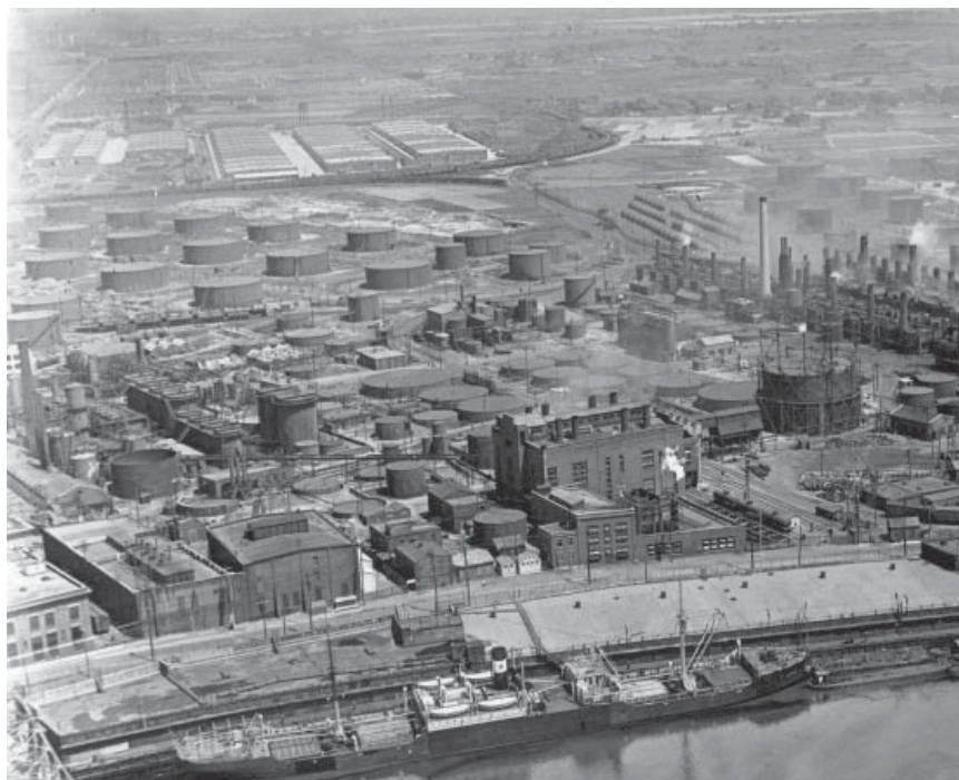
Fig. 3. Atlantic Refining Company's south yard, ca. 1920. This view to the east shows Atlantic Refining's shipping wharf along the Schuylkill River in the lower portion of the photo, the crude distillation stills (each still with its own stack) along the right edge of the photo, the light-fuels treatment area in the left portion of the photo, and petroleum storage tanks in the background. Photo no. P.8990.1861, Aero Services Collection, Library Company of Philadelphia. By permission of the Library Company of Philadelphia.
