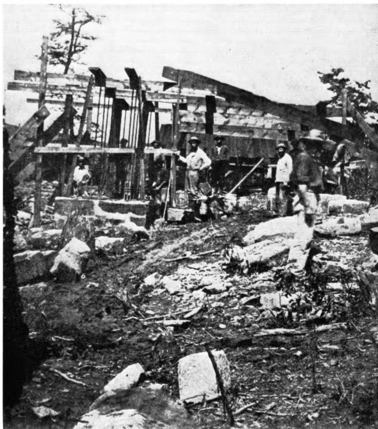
Petroleum Shaft at Petroleum Center, 1866. This was the second attempt to "mine" for oil and was unsuccessful; this is the only known picture of any of the attempts to mine for petroleum.
