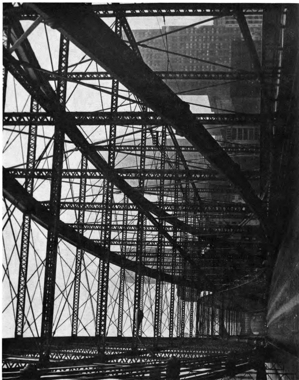
View of the through-trusses of the Smithfield Street Bridge.
