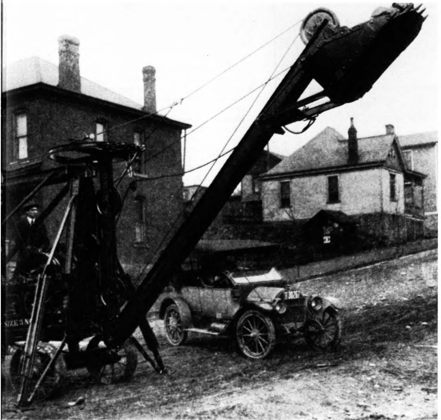
Opposite: A diagram of the sapling technology that Keystone's steam-driven drilling units replaced in the late 19th century. Above: Earth-moving equipment such as Keystone's steam-operated power shovel (c. 1920) dug roads and building foundations throughout America and Europe.
