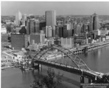
Fort Pitt Bridge under construction, 1958. HHC Detre L&A, Allegheny Conference on Community Development Photographs 1892-1981, MSP 285.
