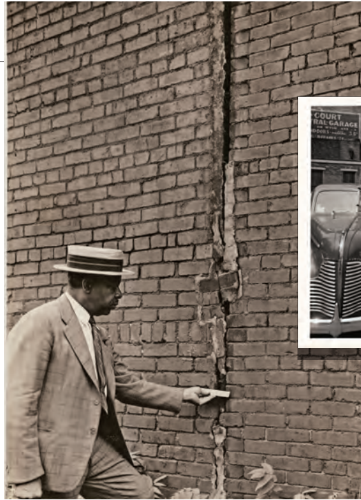
Inspector measuring a crack on a house at 2501 Wylie Ave. in the Hill District, August 16, 1940.
