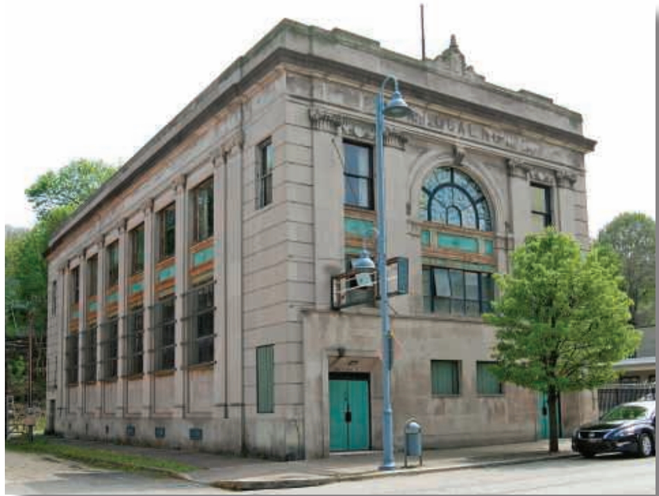
Built as a bank at 501 Franklin Avenue, Aliquippa, in 1927, its frieze proclaims its longtime association with the United Steelworkers Local #1211.
