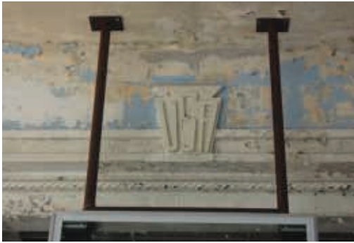
Keystone with the insignia “USA” added by the United Steelworkers of America to the proscenium around the stage in the space of the former bank vault.
