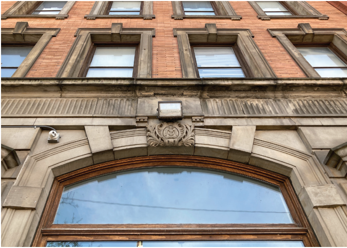
The stone pediments over each first-floor window feature reliefs of the Great Seal of the United States upon cornucopias overflowing with coins.
