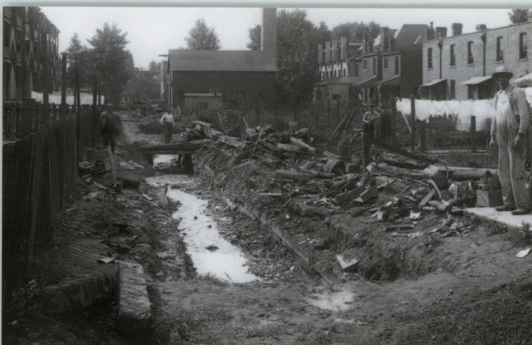
Condition of old wooden drain on Smith Way and damage due to flood, 1911 Collection of STUDIO for Creative Inquiry
