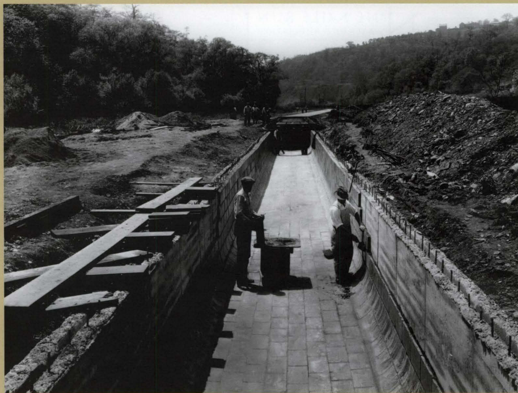
Workers construct a culvert in Nine Mile Run, 1931. Collection of STUDIO for Creative Inquiry
