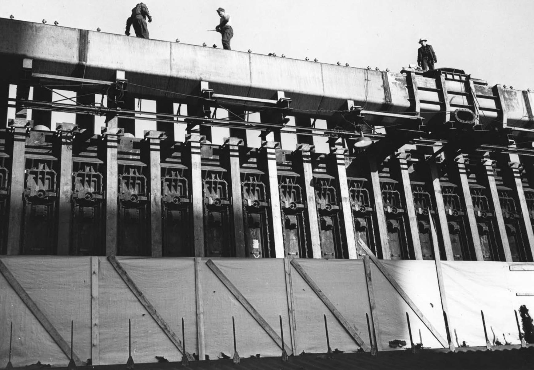
A shift in the battery where coal, 16 tons of it, heats up to 2,000 degrees in fuming ovens just might be a coke oven worker-turned-minister's memory of hell.
